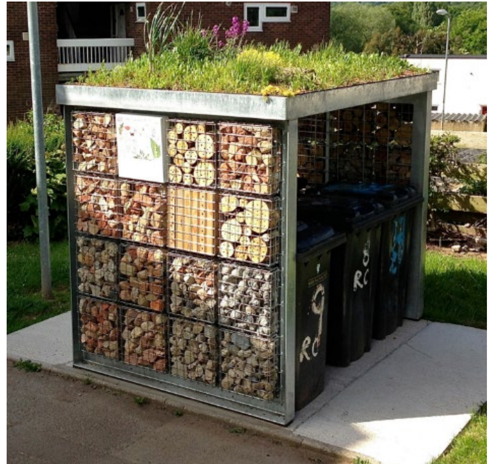
Plate 11: Bin store with green roof and habitat features. Credit: Green Roof Shelters
