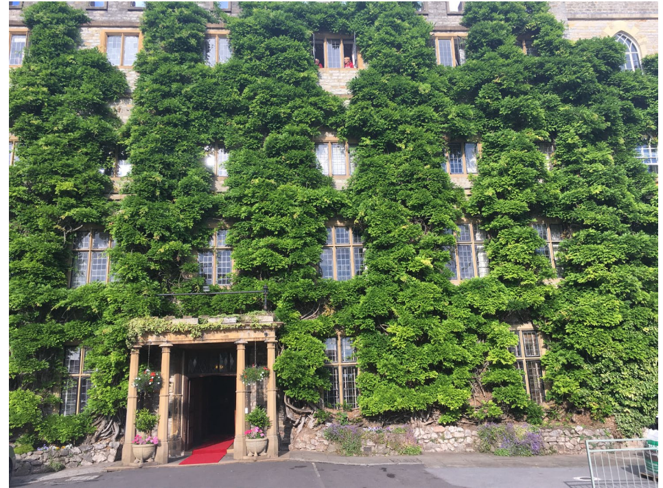
Plate 5: Extensive green wall with climbing plants. Credit: Green Infrastructure Consultancy
