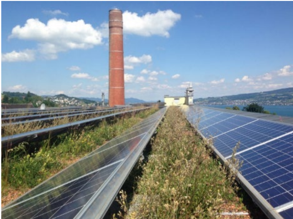
Plate 3: Biosolar roof. Credit: Green Infrastructure Consultancy
